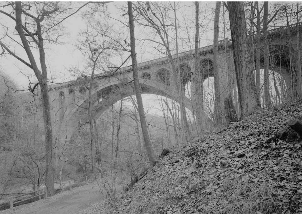
Walnut Lane Bridge, 1998. Historic American Engineering Record, Library of Congress.
